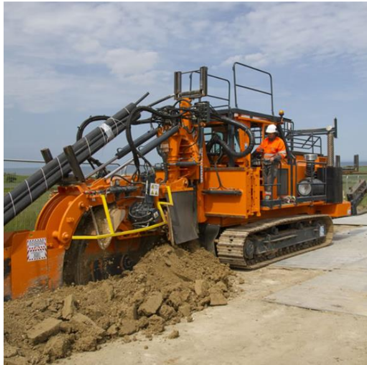
Plate 4-21: Example of cable trenching machine (Source: Equinor)
