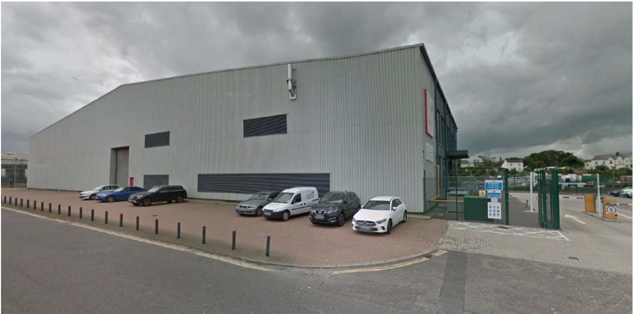
Plate 4-11: Existing SOW and DOW O&M base at Great Yarmouth (Source: Equinor)
