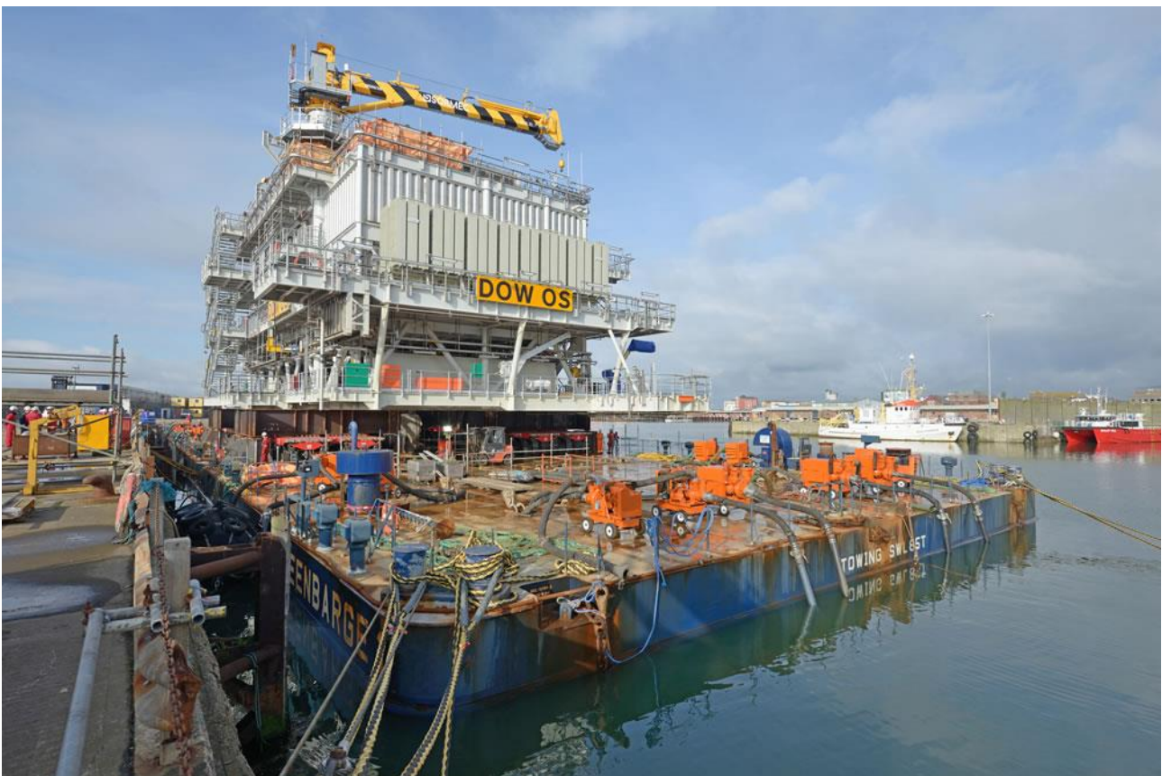
Plate 4-7: DOW OSP being mobilised for installation (Source: Equinor)
