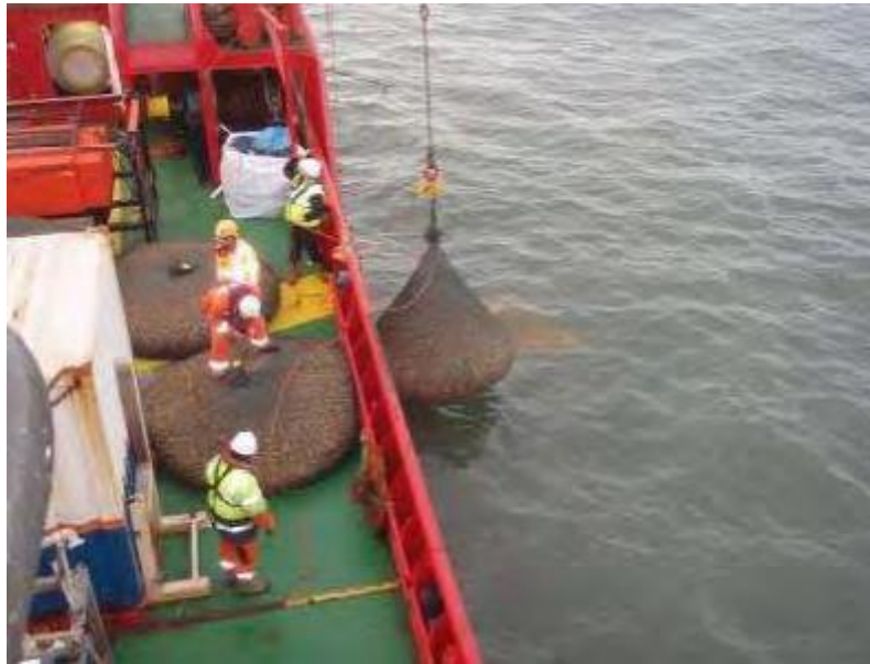
Plate 4-15: Rock bag installation (Source: Equinor)
