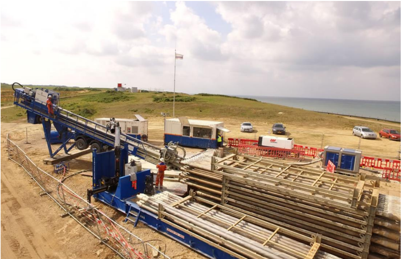
Plate 4-12: Example of an onshore landfall compound (DOW) with drilling rig (left of shot) in operation (Source: Equinor)
