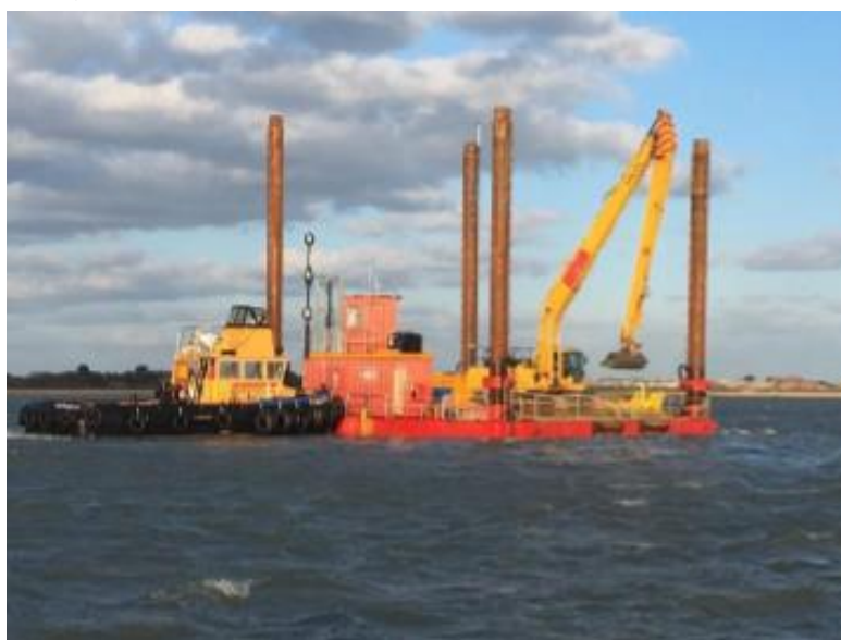
Plate 4-16: Example of a jack-up barge with backhoe excavator (Source: Equinor)
